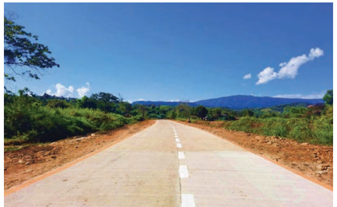
Paving (0/4) miles concrete on the Putao-Laemalwargyi-Namshalkaw- Mansaykhun-Mansay road in Putao Township
