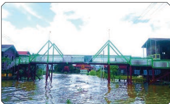
Construction of wooden bridge, Nanhu village in Nyaungshwe Township
