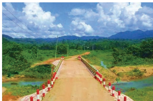
Construction of 100 feet bridge in the entry of Thwaysanyan village in Waingmaw Township
