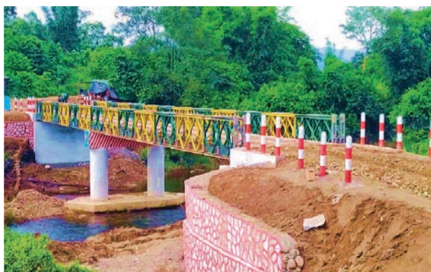
Construction of 130 feet bailey bridge on the access road of Lantaung-Naungkhing village in Putao Township
