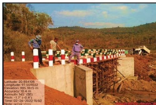
Construction 35 feet concrete bridge on (7/4) miles Namtsan- Naungbo road in Namtsan Township
