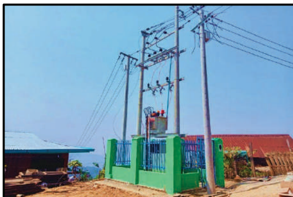
Installing of transformers in Hwaysan village, Sahaung village tract in Loilem Township
