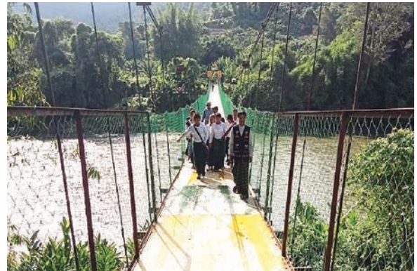
Completion of 360x6 feet suspension bridge in Nanyoon Township
