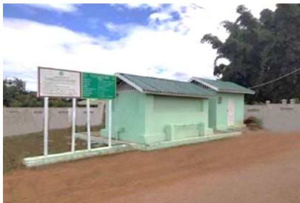
Digging deep tube well in Lashio Township, Northern Part of Shan State
