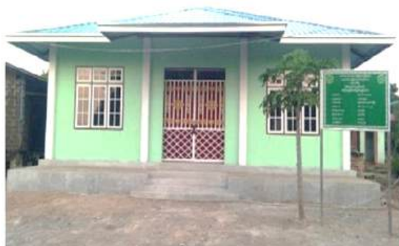
Construction of Community Hall at Thamahta village, Pinlaung Township, Pa-O Self-Administered Zone
