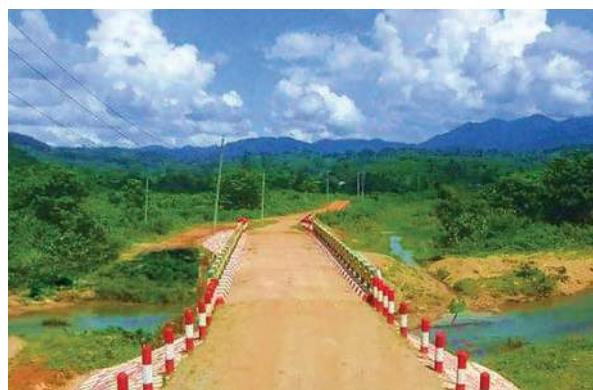
Construction of 100 feet bridge in the entry of Thwaysanyan village in Waingmaw Township
