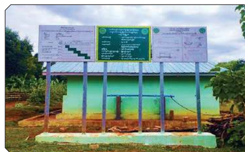
Implementation of Gravity Flow Activities in Tangyan Township (Spring Source)
