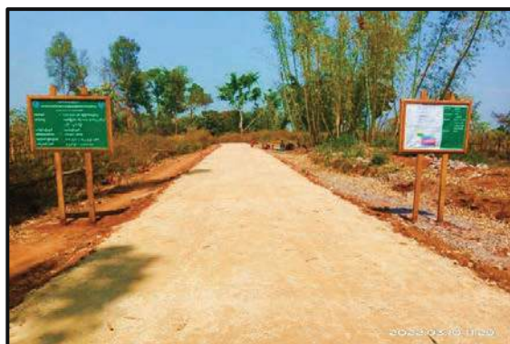
Paving (1/0) miles gravel road among 4 miles on WanPhee-PharLaw-Pansal village, Kyethi Township
