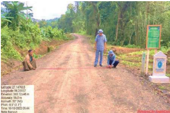
Completion of 3/0 miles maintenance of gravel road in Nanyoon Township
