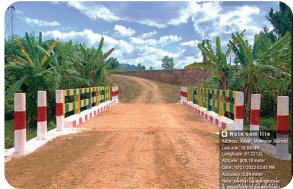
Construction of 25 feet bridge Pain chit village tract, in Loikaw Township
