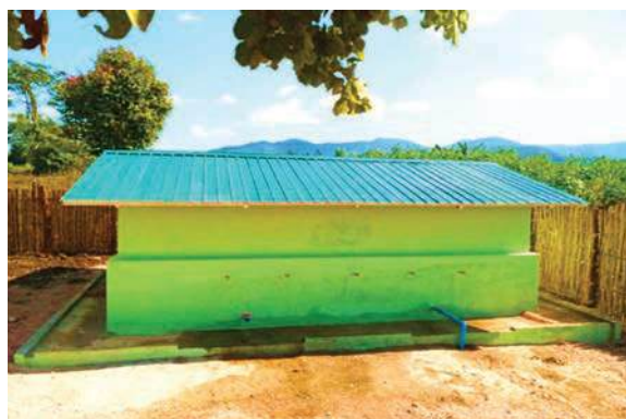
Construction of 10000 gallons brick tank in Lisue village, in Moenae Township
