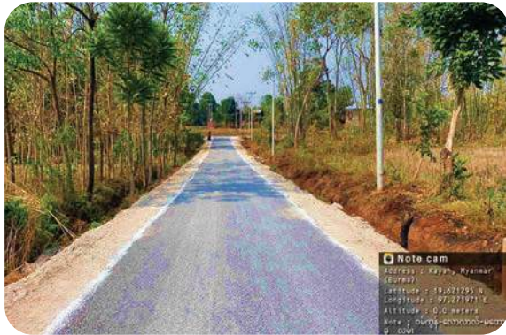
Paving of Nanfe-Tawkuu-Kaykaw road of Thothipho village tract, in Hpruso Township
