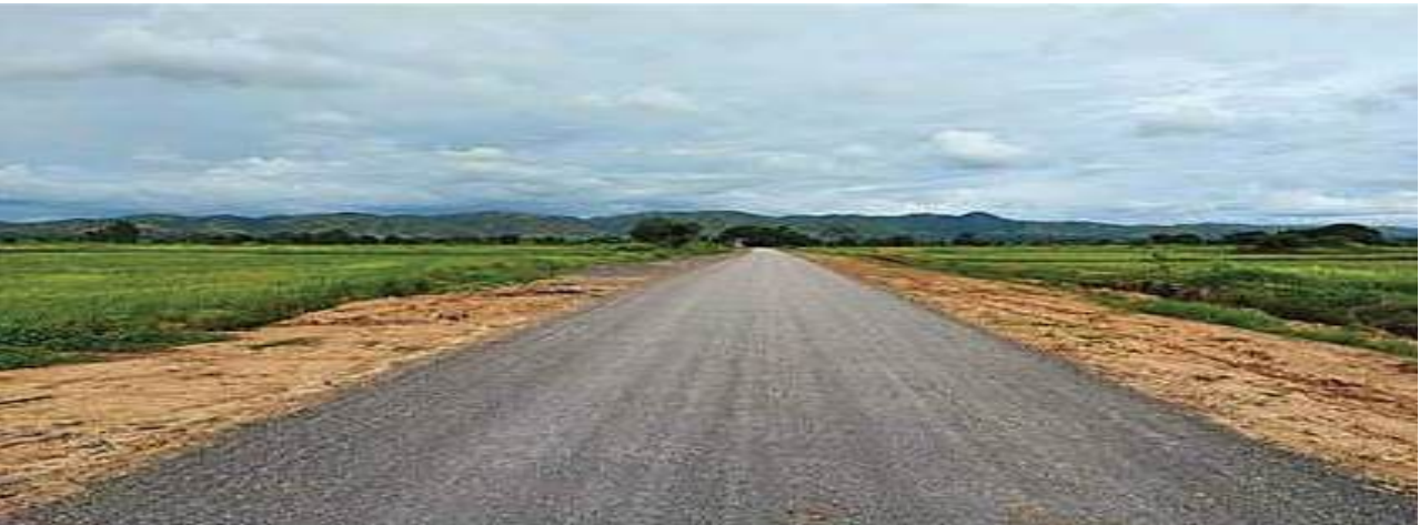
Paving the bitumen road from Main Road, Ywartaw-Myatsat(south)-Myatsat(North)-Bawnanywarthit in Kalaw Township
