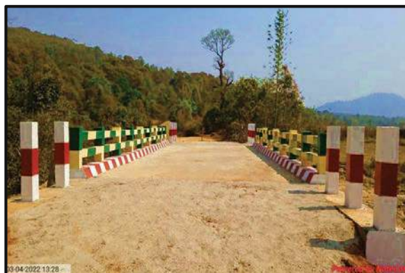
Construction of 40 feet concrete bridge on Kaungsan-Wannaug village tract in Lelchar Township
