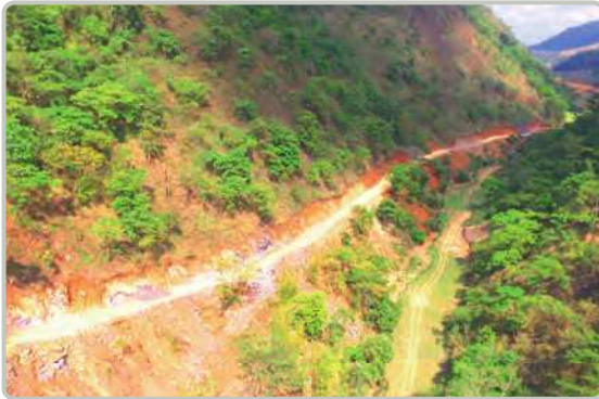
(2/0) miles of gravel road at Khupra-Bardo-Sesaung in Demawso Township
