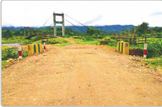
(5) feet Box Culvert on (1/4) miles of Namhtwalkhu gravel road in Putao Township
