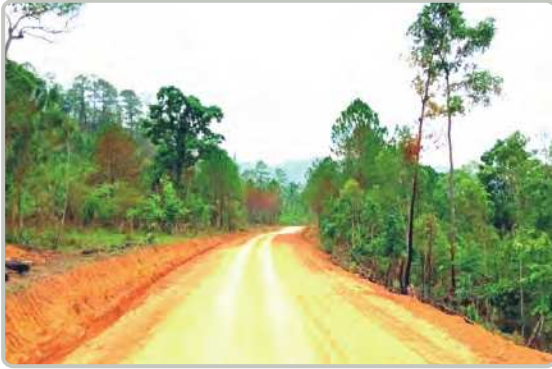
(2/4) miles of earth road at Mineyulay-Gyonenaw-Shoutpangkone-Monewee in Kutkhaing Township
