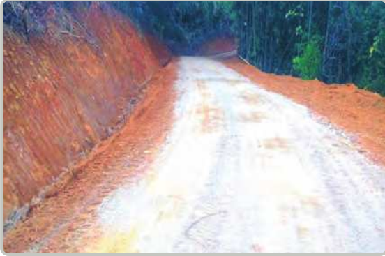
(2/0) miles of gravel road at Pheemaw-Kannphant-Lansal road in Chiphway Township
