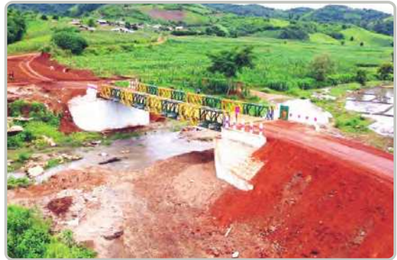
(40)feet of Bailey bridge on (4/4)miles from the center of Mongpan Village to the button in Mongpan village tract, Kyaingtung Township
