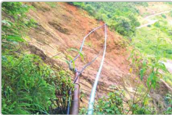
Installation of (11/0) miles damaged water pipeline in 4 quarter of Tedim Township
