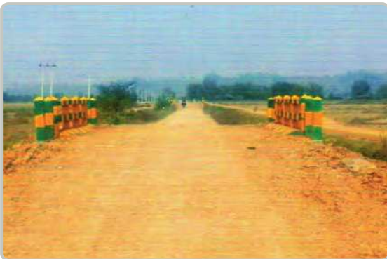
Concrete bridge on Magweza-Kaung Lan Phu road in Khaung Lan Phu Township
