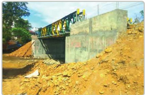
(50) feet of Bailey bridge at Marmeim-Marmeim Sheedee Village in Putao Township
