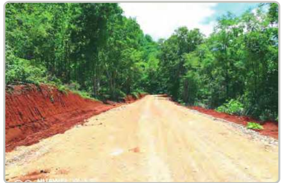
(3/7) miles road extension at Hoyar-Rikeebue-Kharbal-Bwaldoe in Hpruso Township
