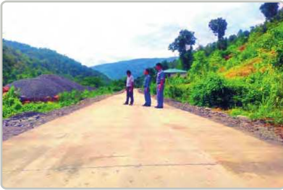
(2/0) miles of concrete road at Khaingkam-Painpi in Tedim Township
