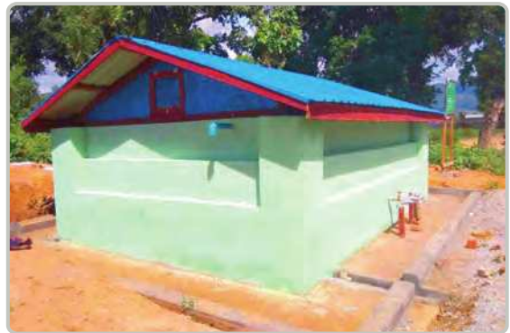
(5000) gallons pond at Township Supervisory Office in Tonzang Township
